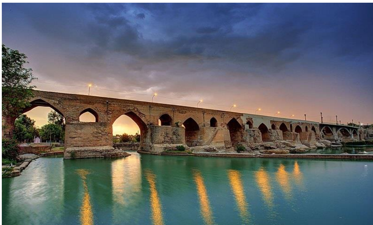
Old Bridge of Dezful
